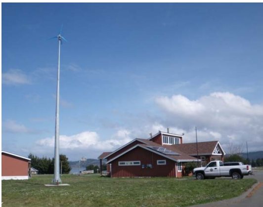
1500 Watt wind turbine on a 45 foot tower, and 2100 Watt solar array mounted on the Community Center roof
