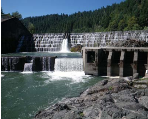
Figure 1. Van Arsdale Dam with fish ladder (box structure on right)
